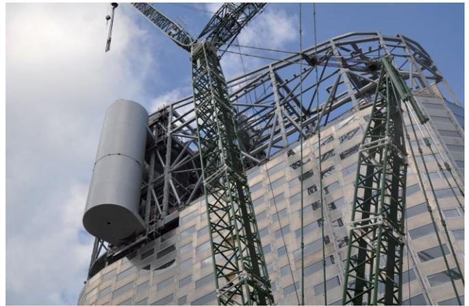
Fig. 16. Lifting unit 2 of the chimney (by Züblin Stahlbau)
