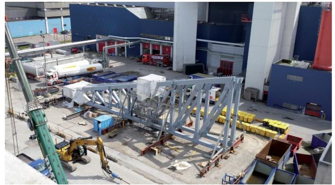
Fig. 5. Preassembled truss for waste bunker (by Züblin Stahlbau)
