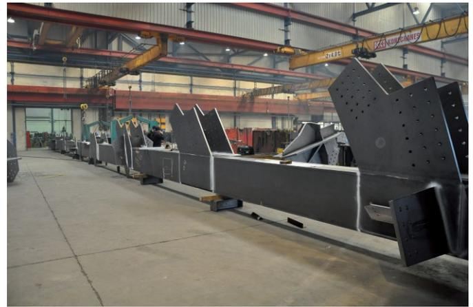
Fig. 11. Preassembly of the 40 m long truss chord for waste bunker in fabrication shop (by Züblin Stahlbau)
