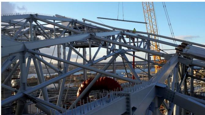
Fig. 7. Upper chords of roof trusses for process building (by Züblin Stahlbau)
