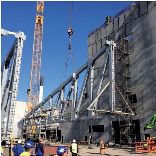
Fig. 13. Lifting the first truss for the waste bunker (by Züblin Stahlbau)
