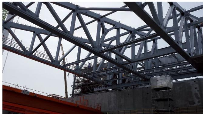
Fig. 12. Intermediate construction step of the roof trusses for the waste bunker (by Züblin Stahlbau)
