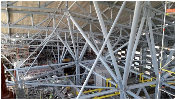
Fig. 4. Tree-like roof structure for process building (by Züblin Stahlbau)
