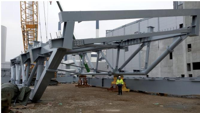
Fig. 14. Lifting a preassembled unit for the process building (by Züblin Stahlbau)
