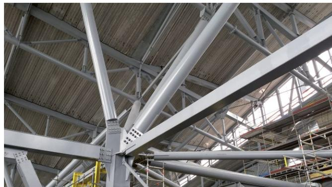
Fig. 8. Column head in tree-like structure (by Züblin Stahlbau)
