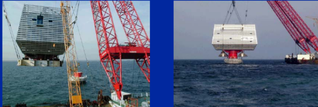
Installation of the SEAS platform
