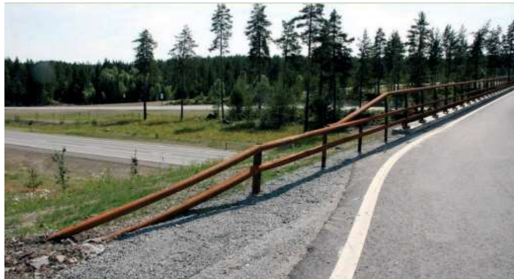
Don't use weathering steel close to roads on which de-icing salt is used
