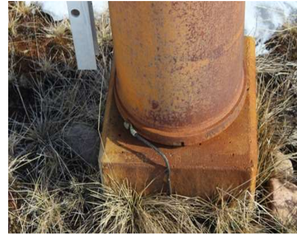
Discoloring of concrete
