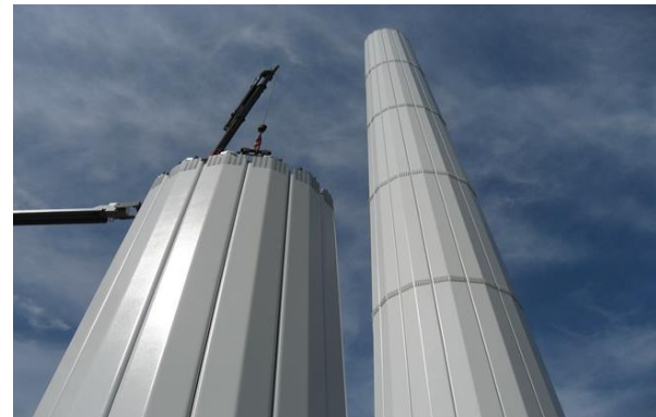
Assembly and installation of bolted steel shell tower sections
