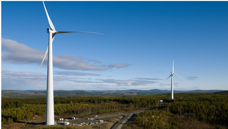
Bolted steel shell tower installed with wind turbine from Siemens Wind Power A/S at Stamåsen wind farm
