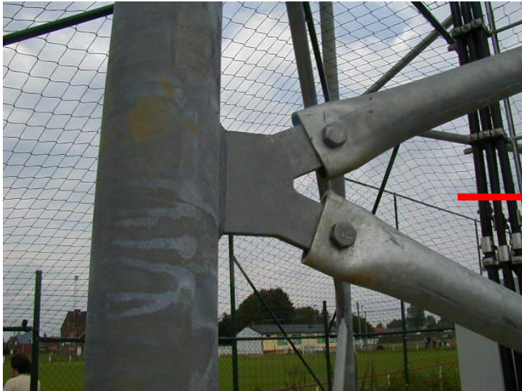
Squeezed bracing joint in telecom tower, Romania
