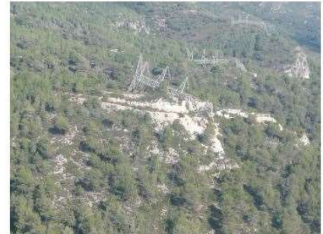
Figure 1-3 Transverse cascade on the 400 kV D/C Rubí-Vandellós-Pierola line in Spain during a 2008 HIW storm. (Photo: J. Santana López)
