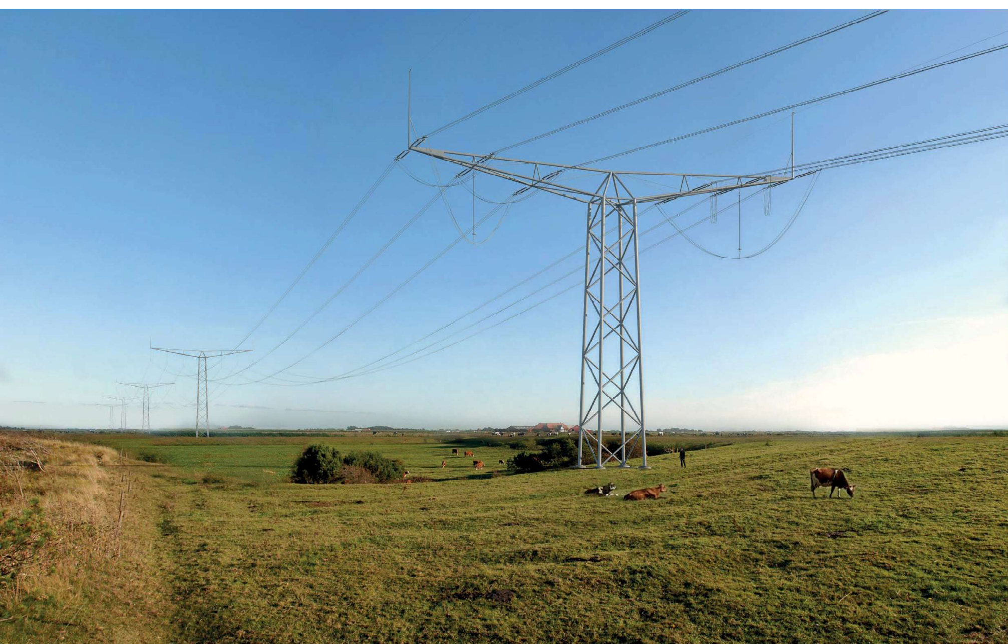
MASTETYPE FASETRANSPONERINGSMAST (0°), illustration (24 METER)
