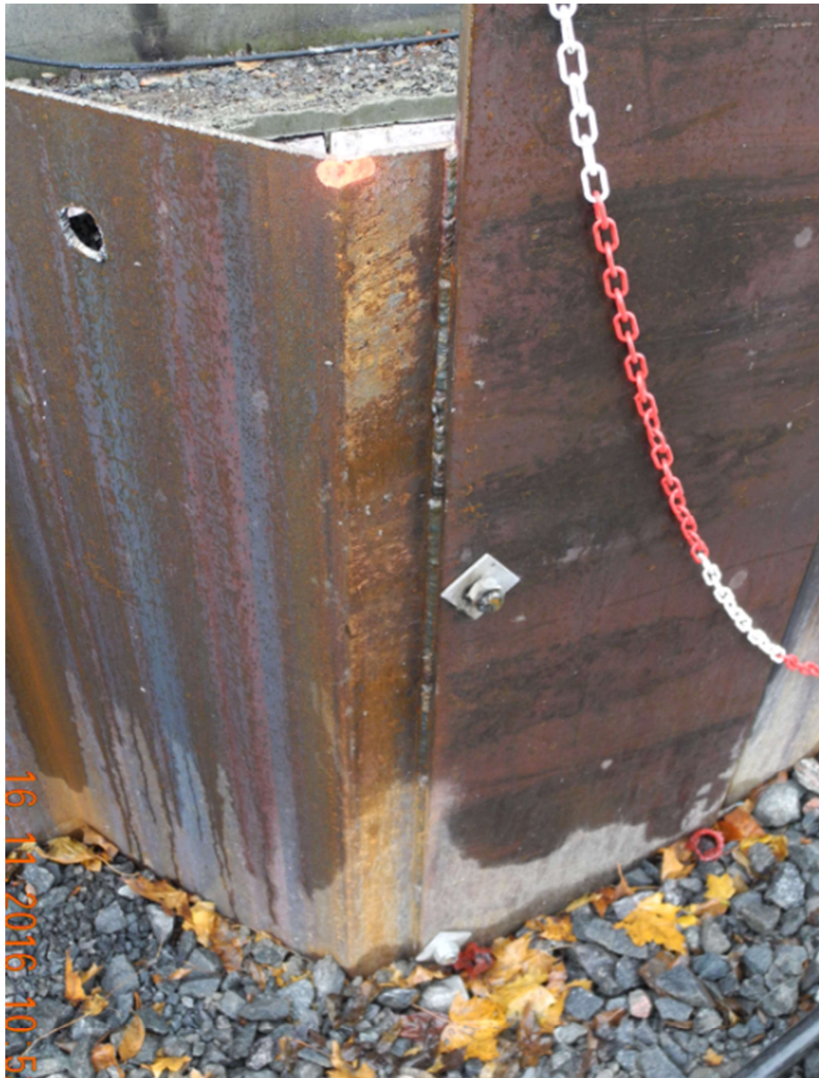
Special pile fabricated on-site
