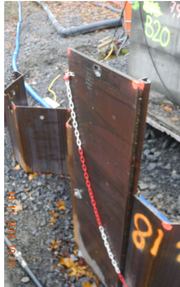
Special pile fabricated on-site
