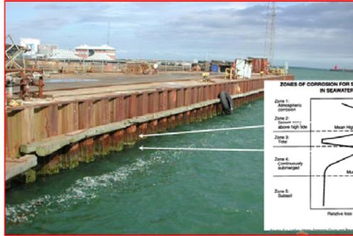
**ZONES OF CORROSION FOR STEEL PILING IN SEAWATER**
