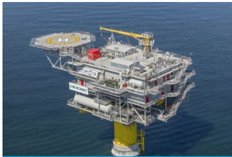
Substations HVAC / HVDC
