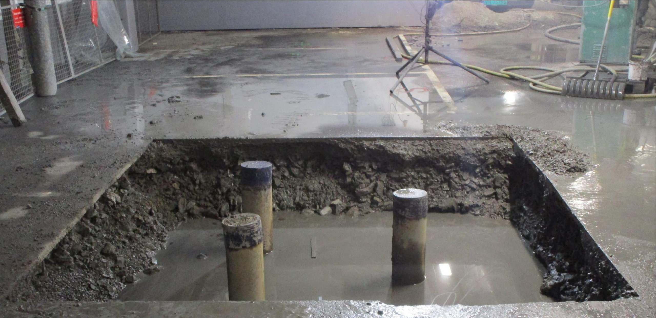
Karenlyst Allé, Oslo – RD micro piles (underpinning)
