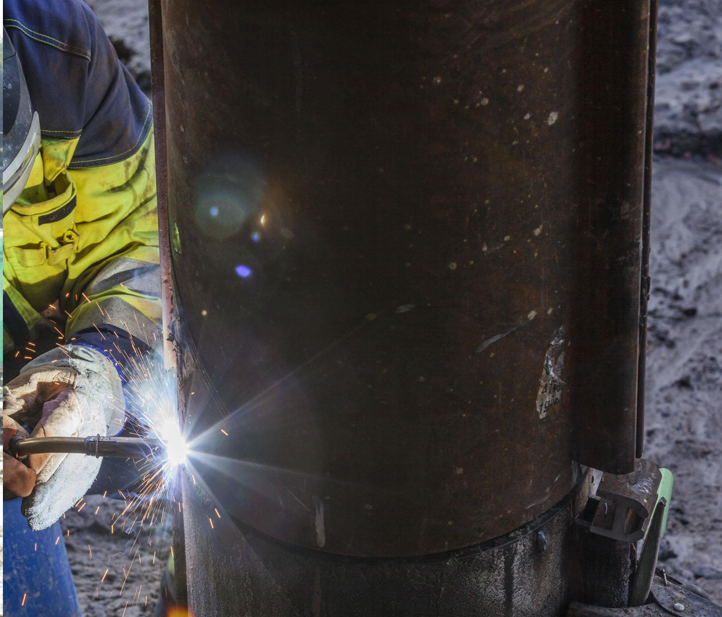
Splicing at site – RD Pile Wall
