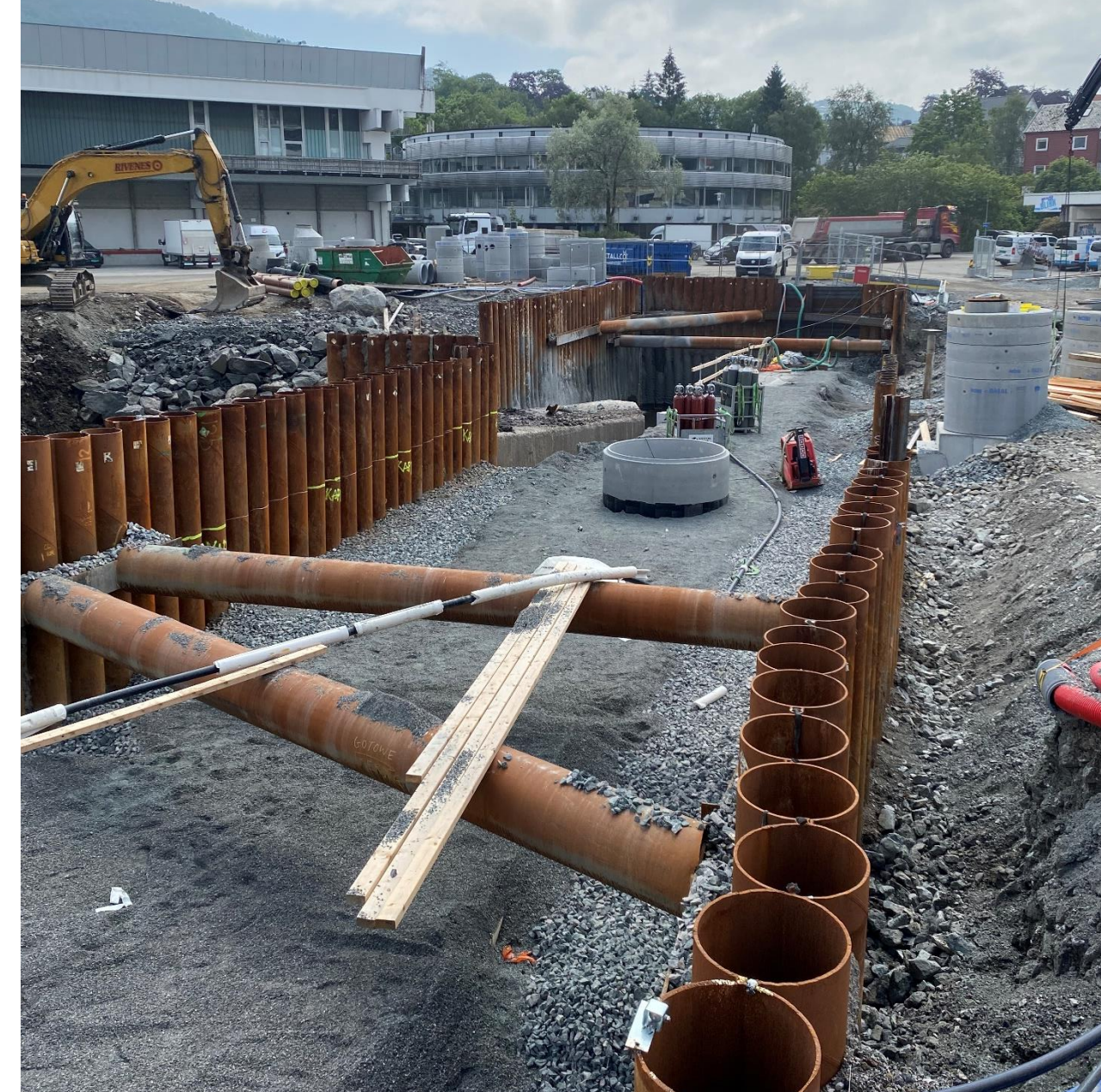
City Tram, Bergen Norway – RD Pile Wall
