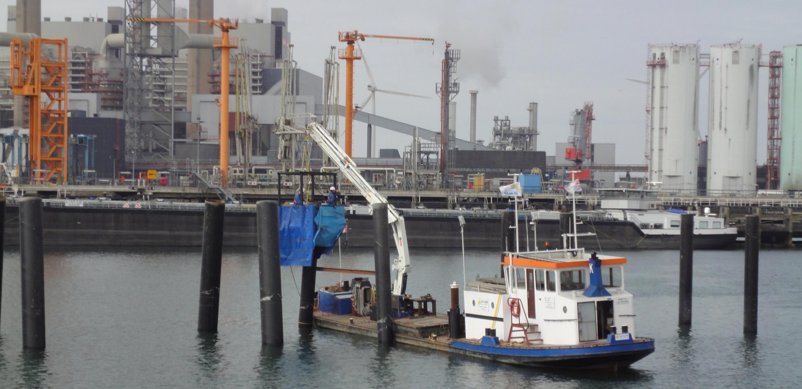
Rotterdam, Netherland – LDP, RR piles w/ PE-coating
