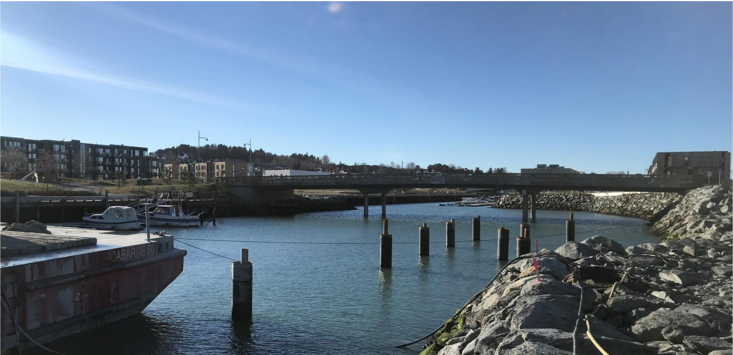
Grillstad Marina, Trondheim – Pipe in pile with PE-coating
