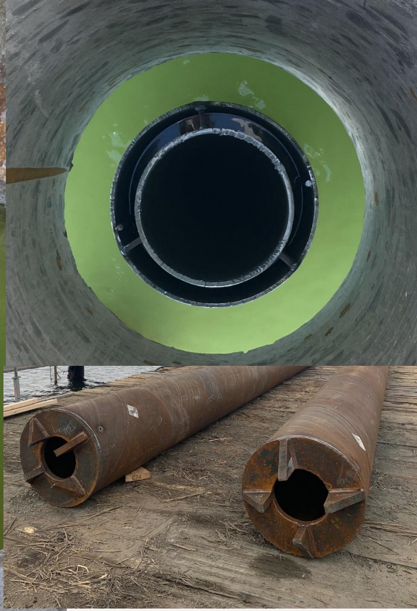
Marine installation in Stockholm – RD micro piles SSAB
