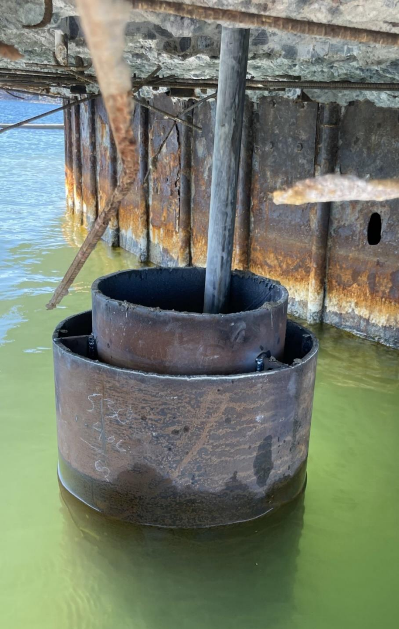
Marine installation in Stockholm – RD micro piles SSAB
