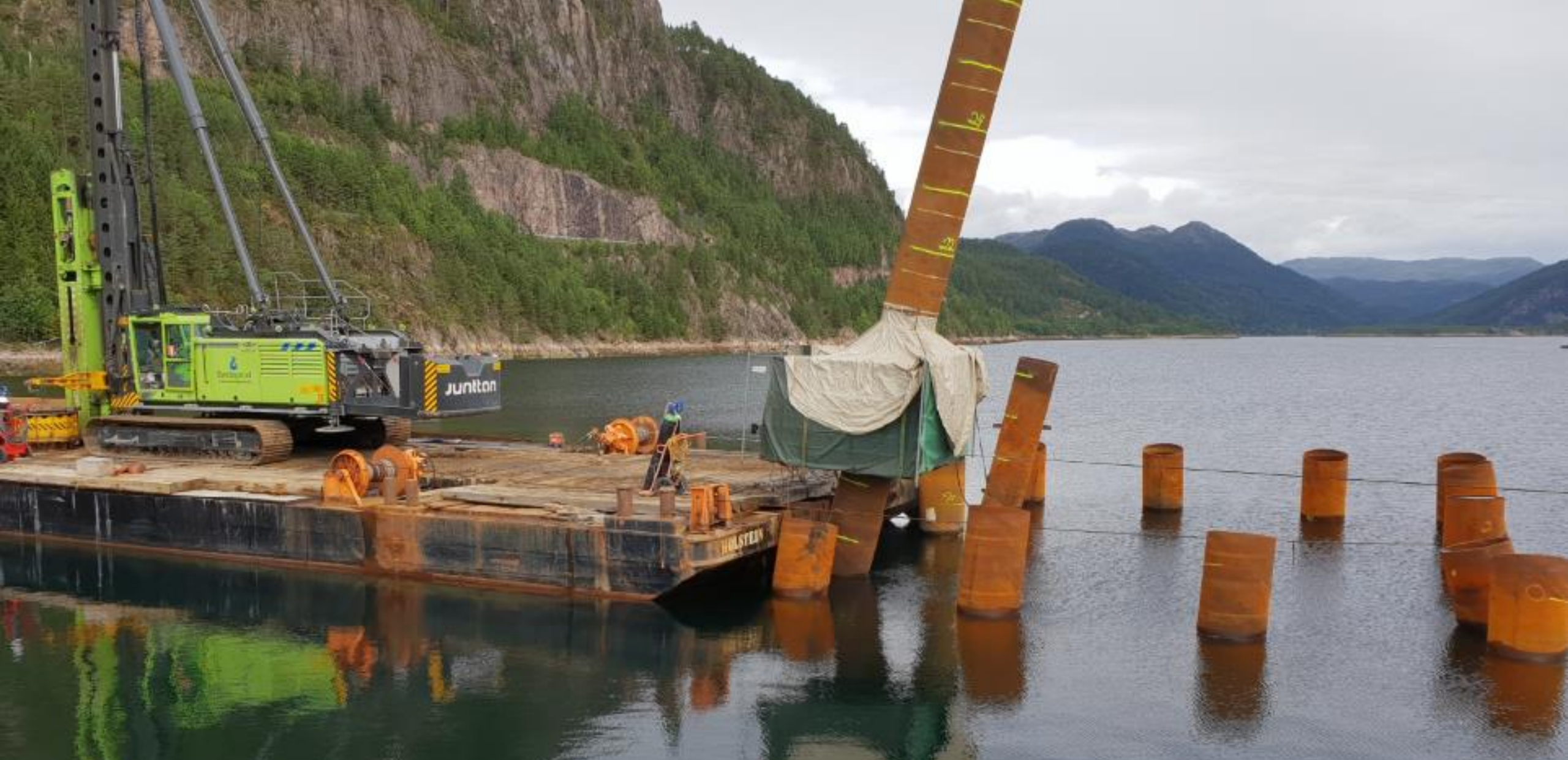
Åstfjorden, Trøndelag – LDP, RR piles
