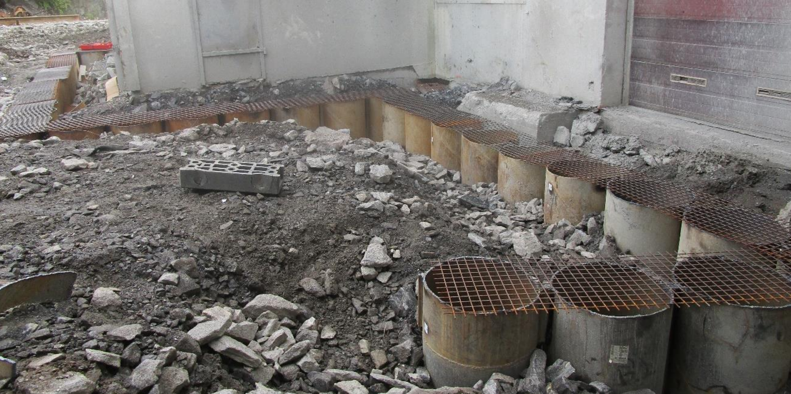
Polluted ground, Bergen Norway – RD Pile Wall
