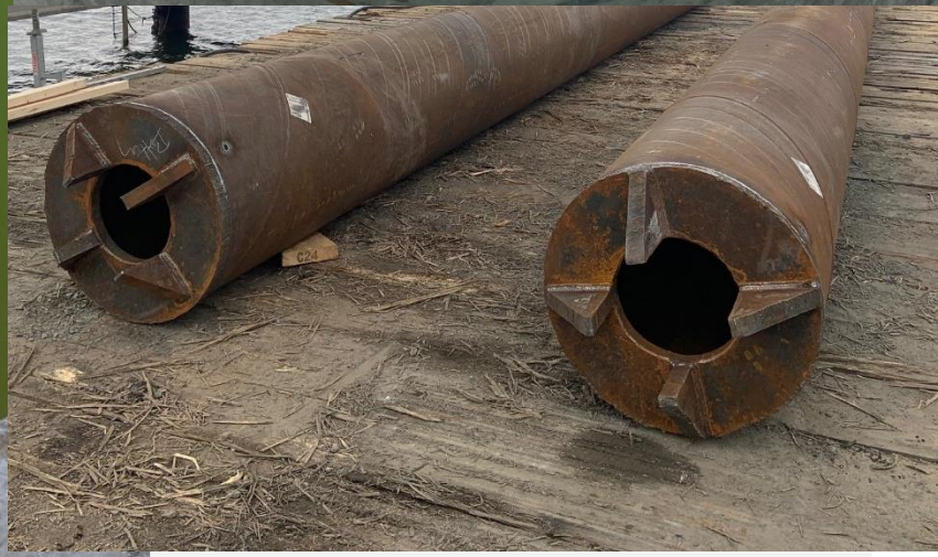
Marine installation in Stockholm – RD micro piles SSAB
