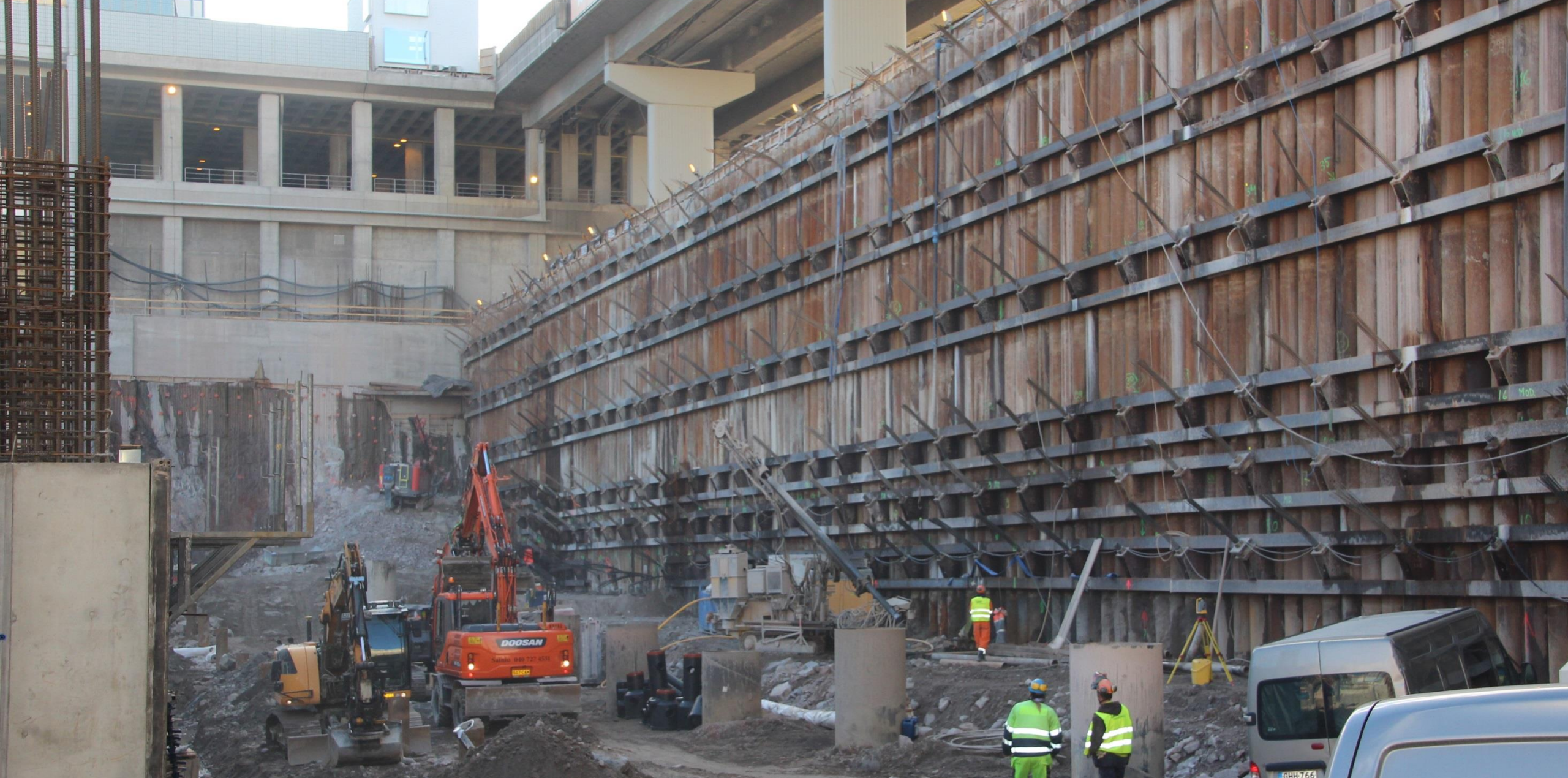
Pasila Tripla, Helsinki Finland – RD pile wall
