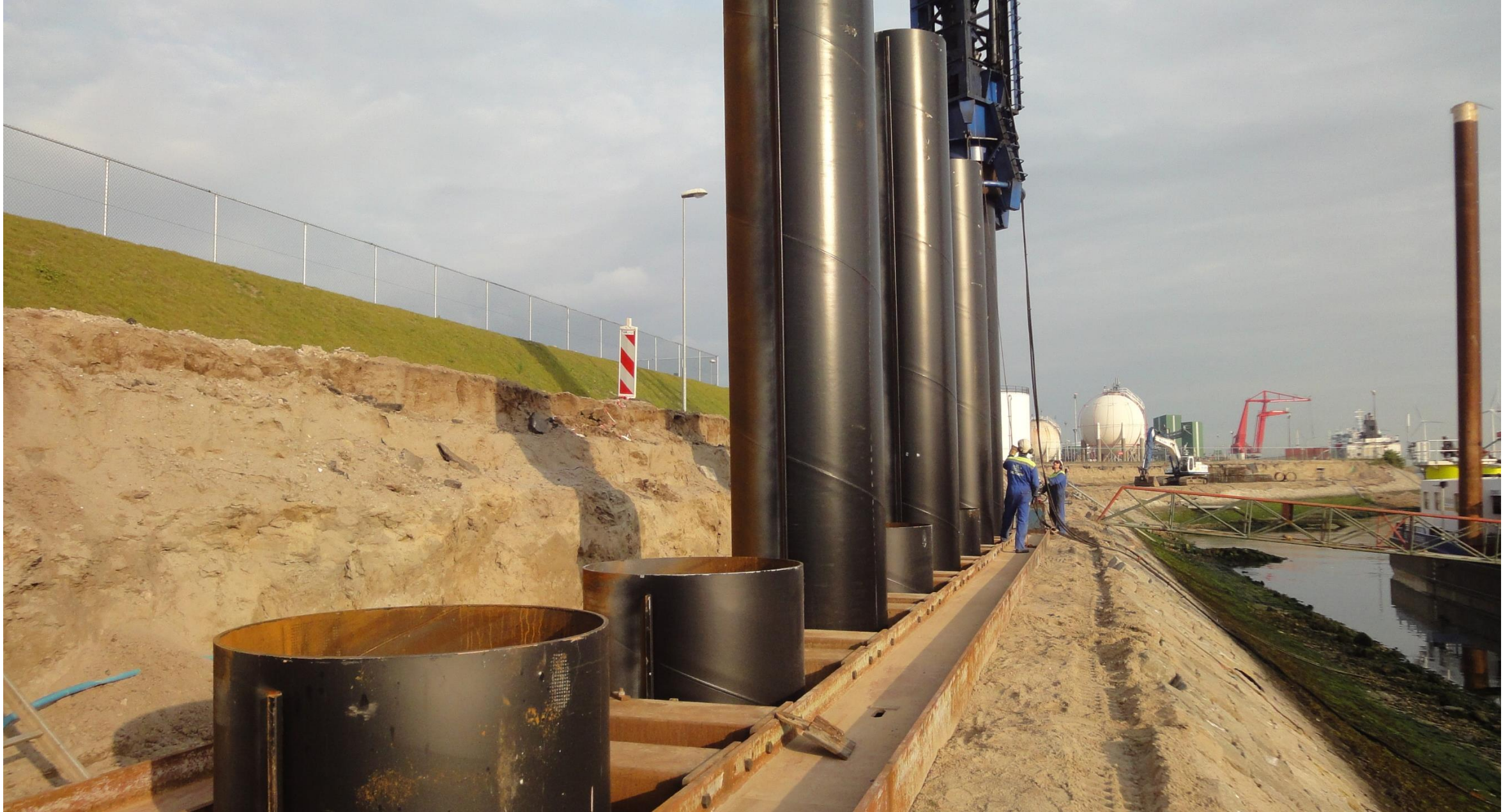
Rotterdam, Netherland – Combi Wall w/painting
