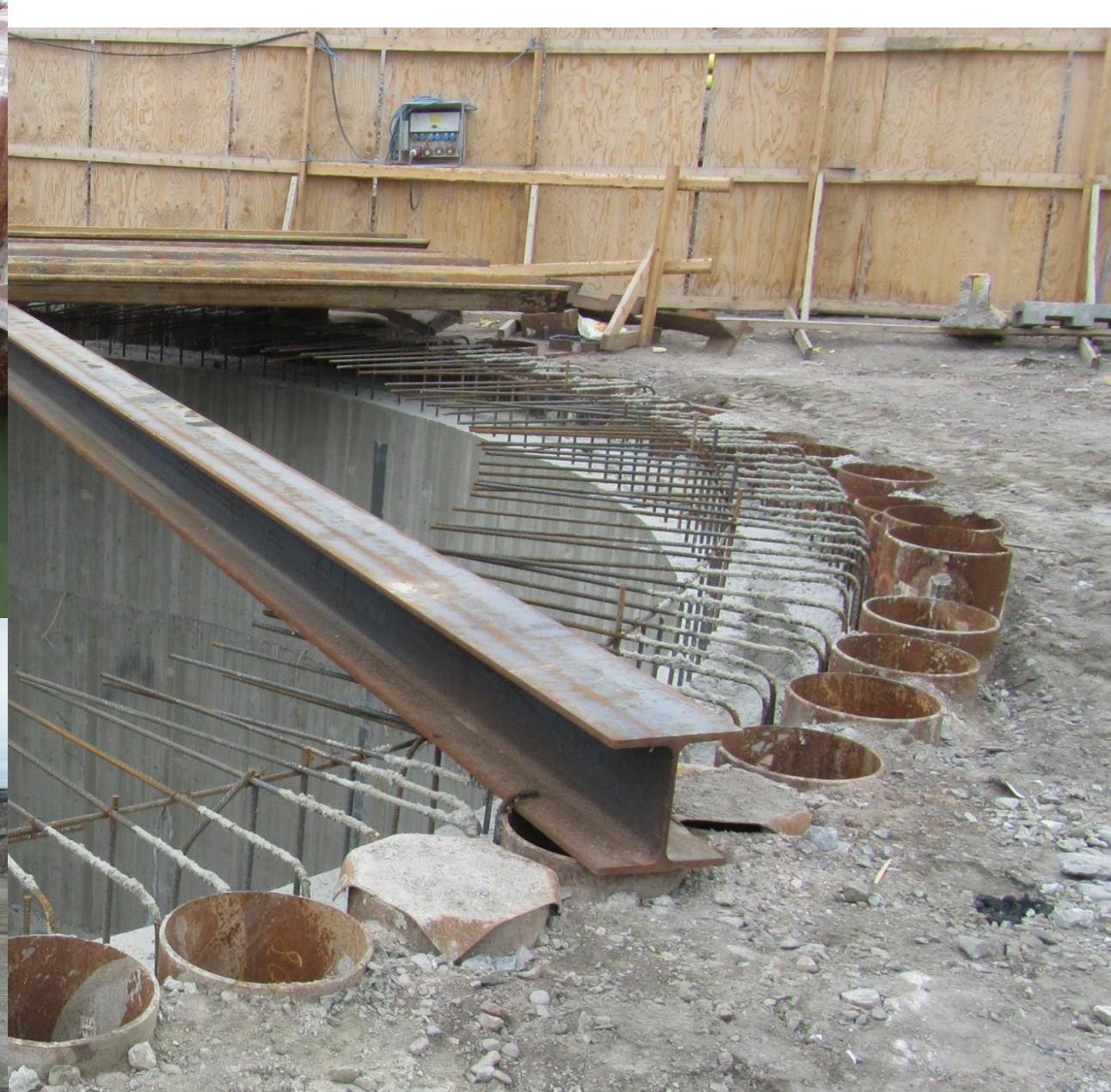
Helsinki, Finland – circular RD pile wall
