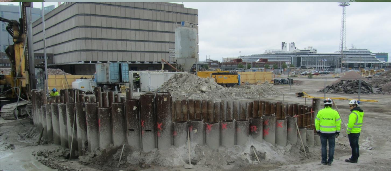
Helsinki, Finland – circular RD pile wall
