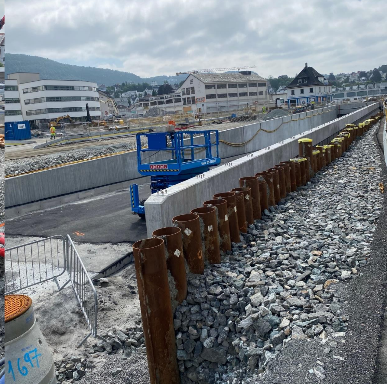
City Tram, Bergen Norway – RD Pile Wall
