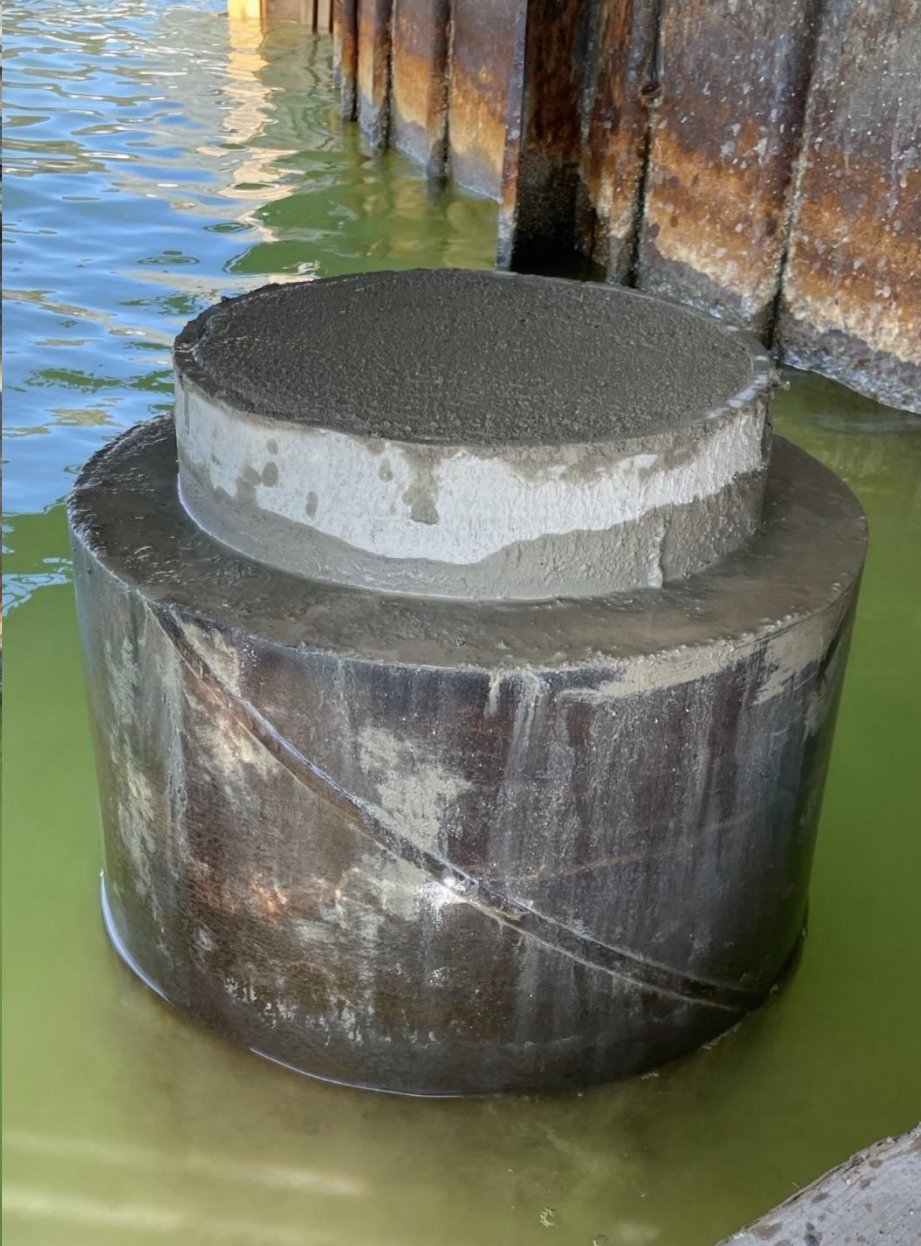
Marine installation in Stockholm – RD micro piles SSAB
