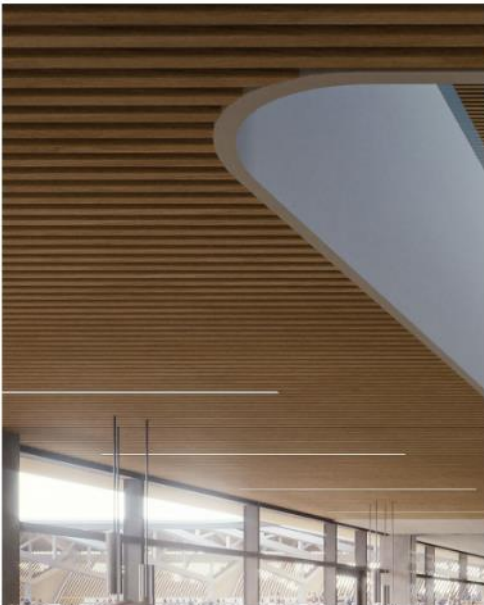
Acoustic Ceiling With Embedded Lighting
